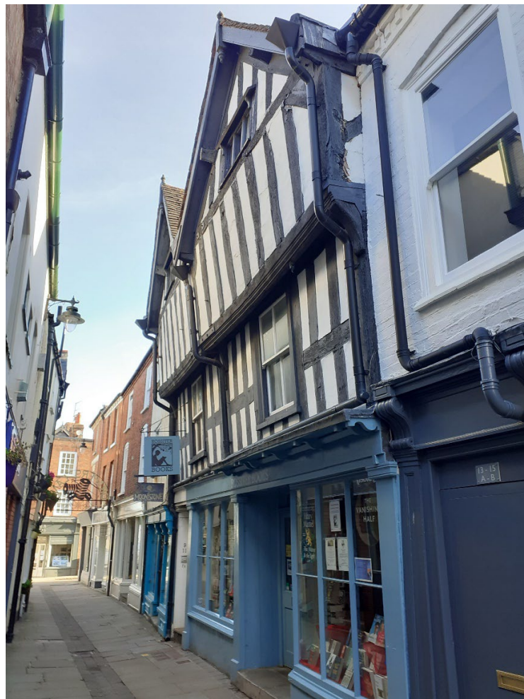
Plate 9: View looking north-northwest along Drapers Lane, showing twin gabled and jettied timber-framed building at Nos. 9-11, of 16 th /17 th century date
