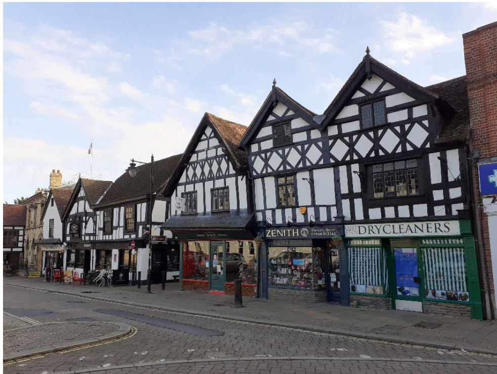
Plate 7: View looking southeast towards series of 15 th -17 th century timber framed buildings along the south side of Corn Square at the junction with School Lane
