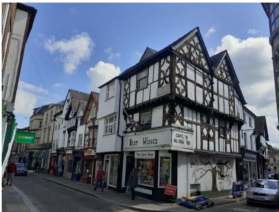
Plate 8: View northeast showing the corner of High Street and Corn Street showing a series of late 16 th /17 th century timber framed buildings including Nos. 43-45 High Street in foreground
