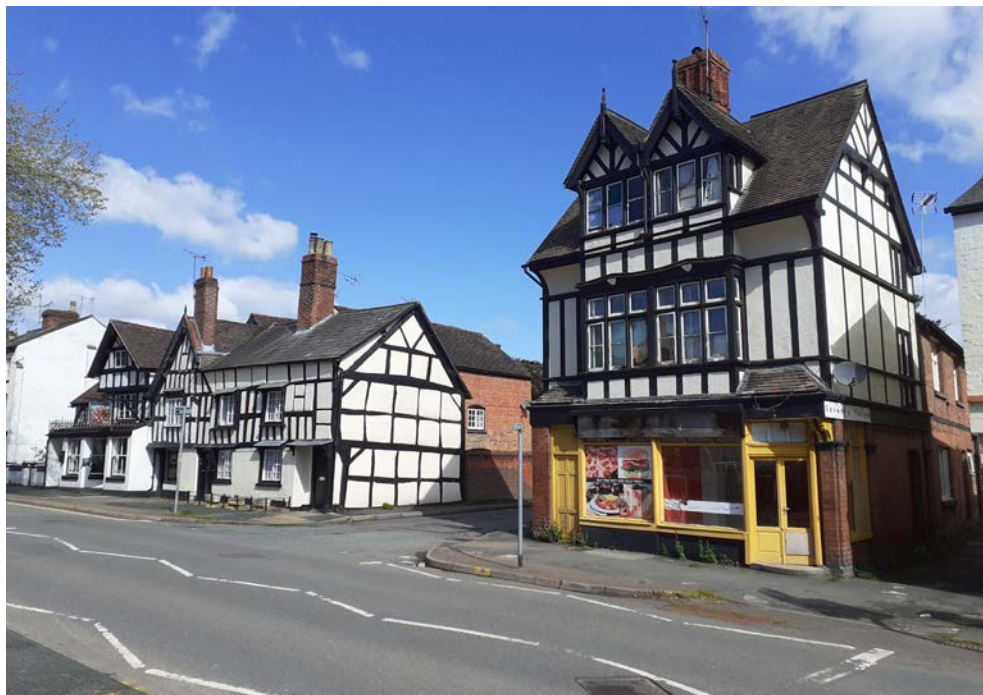
Plate 16: View looking northwest towards the Chequers Inn and Nos. 63-67 Etnam Street (of 16 th /17 th century date) with No. 73, a late Victorian building to right of picture
