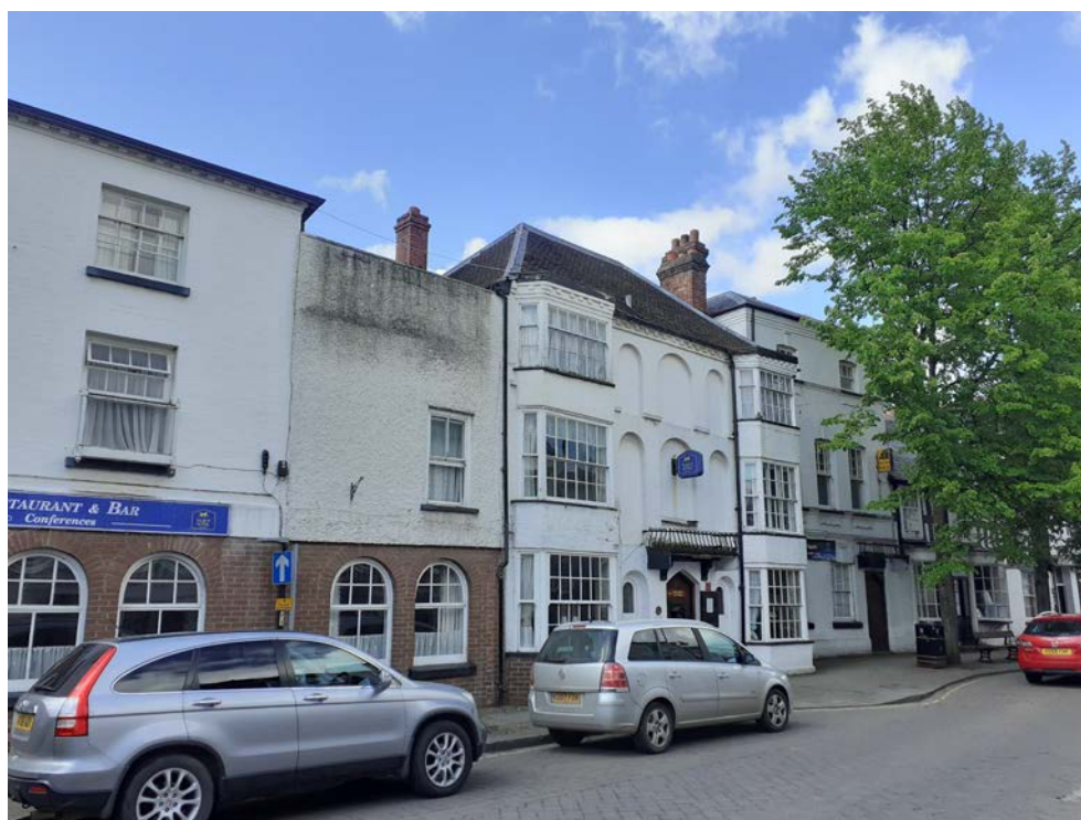
Plate 21: View southwest showing the frontage of buildings comprising the Talbot Hotel
