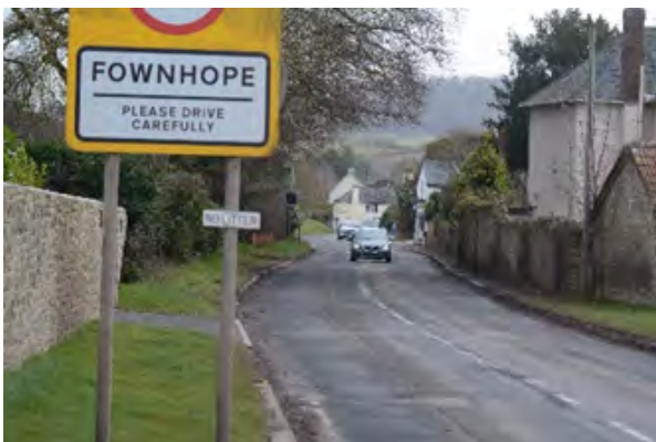
Example 1: Wide verges on both sides with walls set back from the road. The wall on the left is modern but constructed from materials reflecting traditional methods. A traditional wall on the right has a narrow verge between it and the road.
