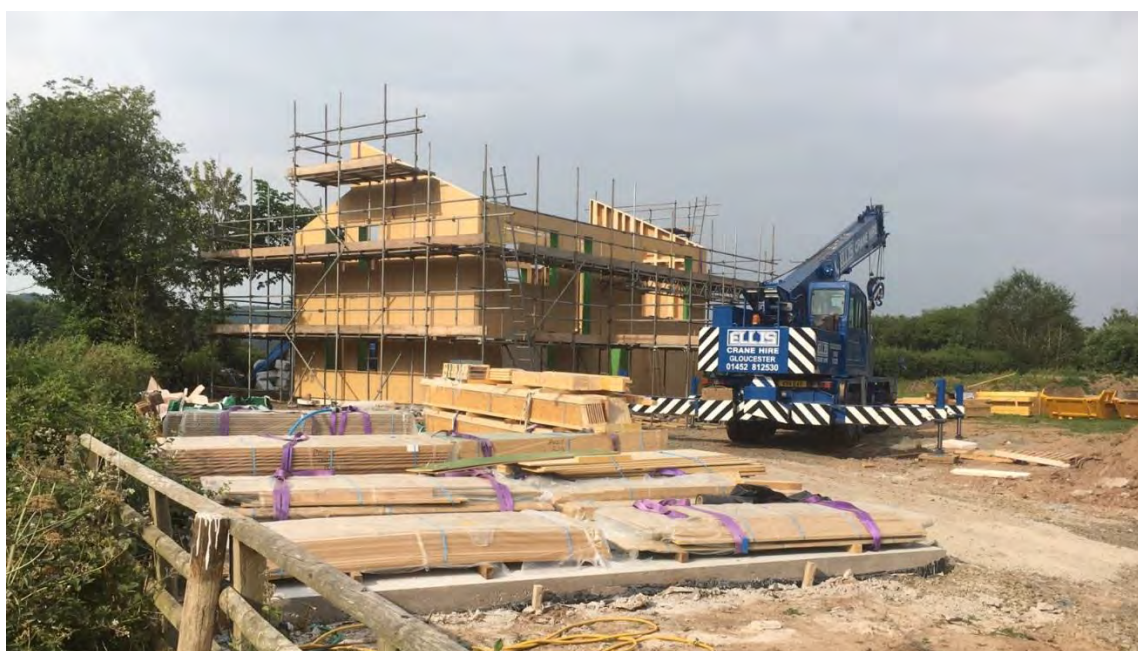
Picture 10: Building an energy efficient Passivhaus in Clifford Village.
