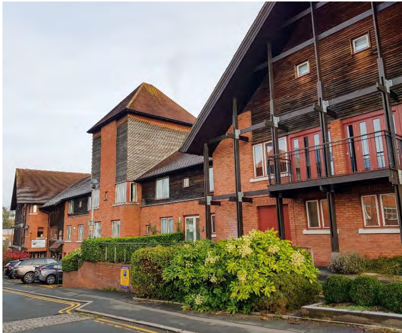
Figure 27 - Ledbury Community Health and Care Services and Medical Centre
