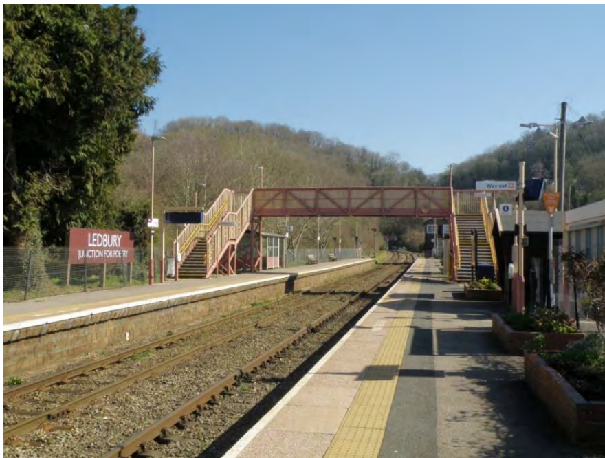
Figure 32 – Ledbury Railway Station
