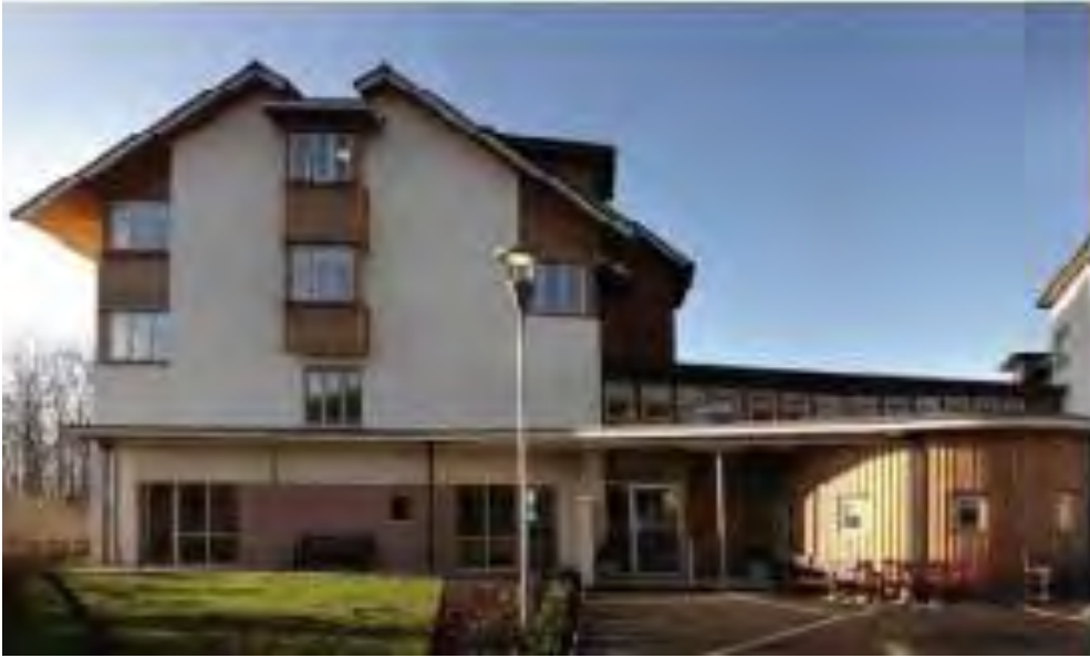
Figure 15 - Leadon Bank Sheltered Housing
