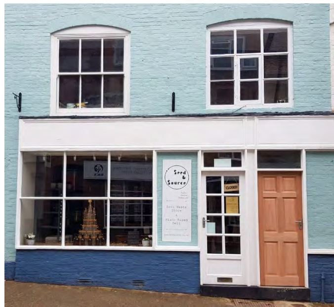
Figure 19 - Shop on New Street
