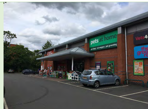
Figure 7: Brook Retail Park, located to the north of the city centre, is a key retail destination in the city centre.
