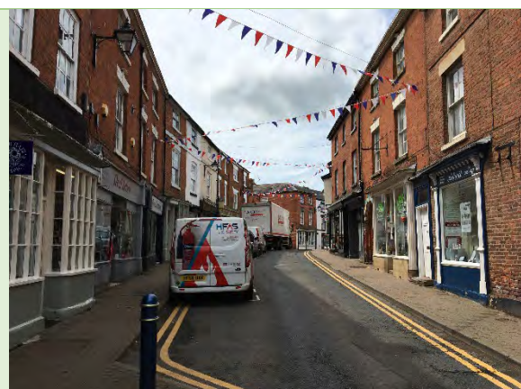
Figure 4: Broad Street and High Street are the main retail parades in Bromyard.
