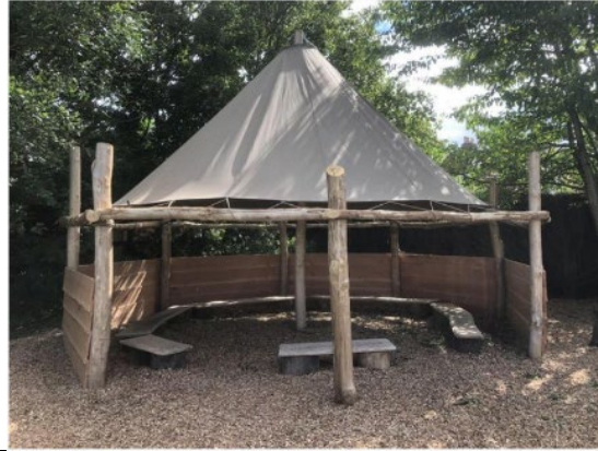
Figure 6 – Delivery of outdoor classroom St Thomas Cantilupe Primary School
