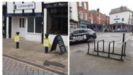
Inappropriate and poorly maintained street furniture
