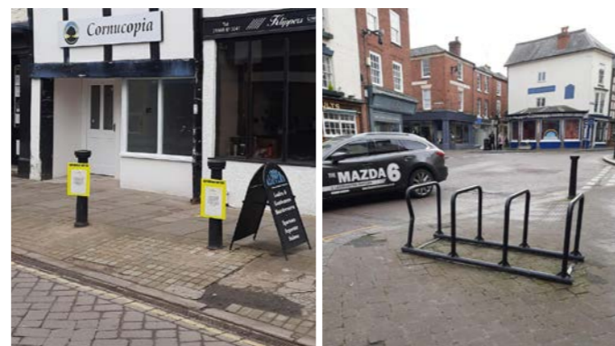
Inappropriate and poorly maintained street furniture
