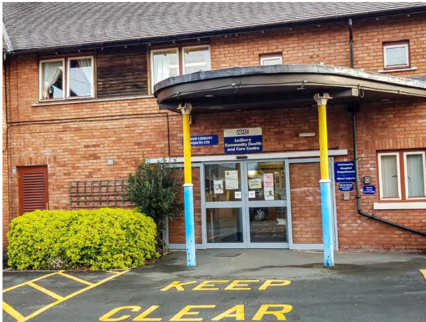
Figure 26 - Ledbury Community Health and Care Centre
