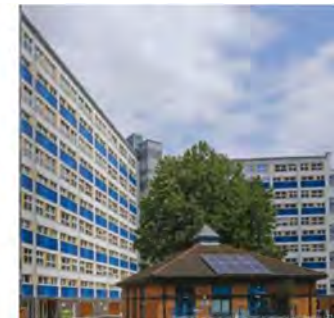
Wilmcote House, Plymouth (Source: ECD Architects)
