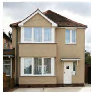
Grove Road, London (Source: Bere Architects)
