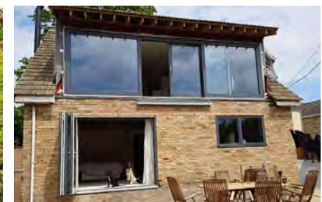
Wholehouse retrofit, Cambridgeshire Source: Green building store
