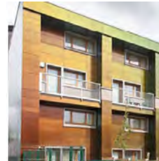
Ernley Close, Manchester (Source: 2e Architects)
