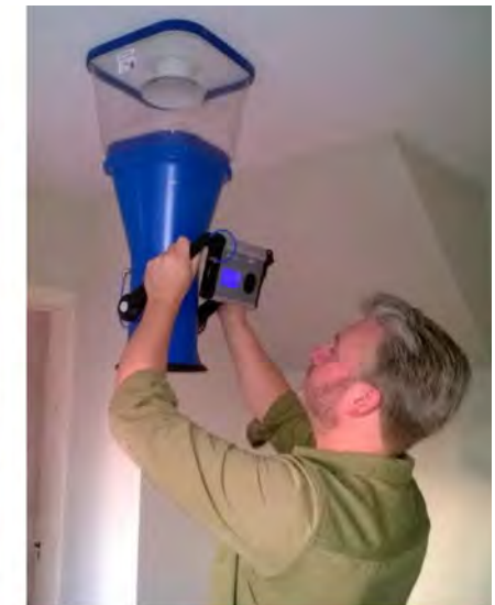
Flow rate measurement: image of MVHR system being commissioned (Source:Fourwalls)
