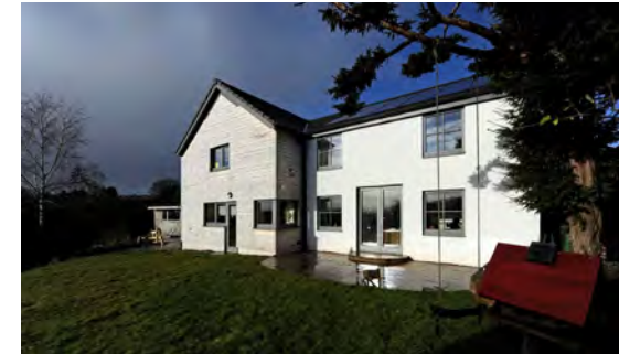
Reform Cottage, Kingsthorne, Herefordshire Source: Andy Simmonds Architect
