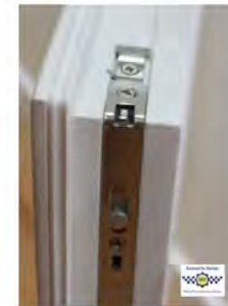
Multi-point locking mechanism (Source: Sashed)
