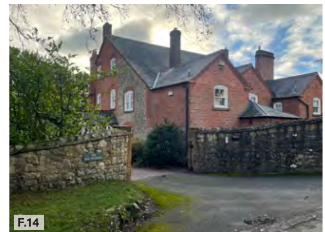
Figure 14: Further examples of red brick and stone can be seen throughout the village.
