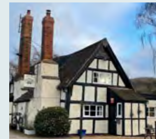
Timber frame with plaster infill
