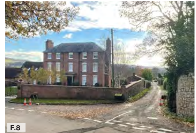
Figure 08: Grade II listed Stone House.
