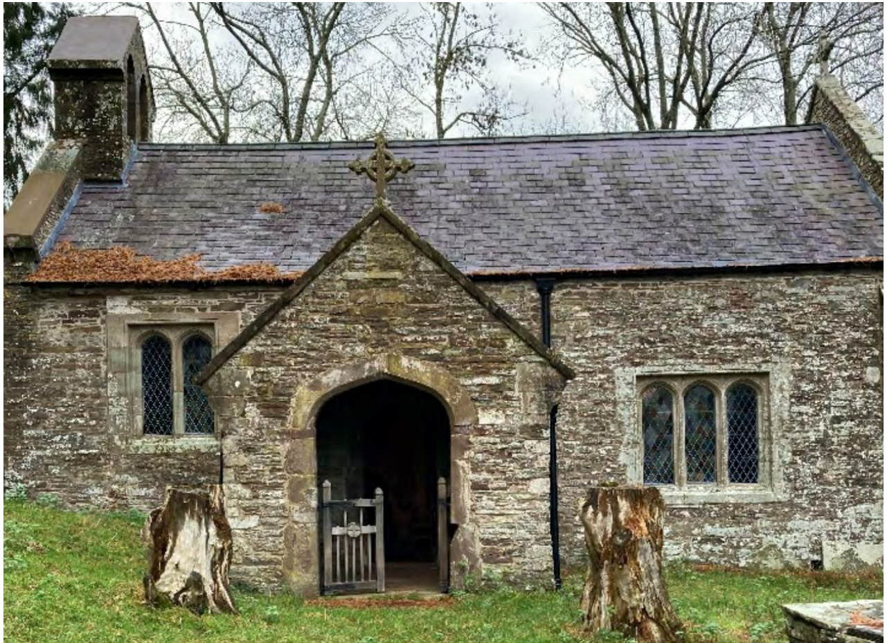
Figure 7.21: Pipe Aston church
