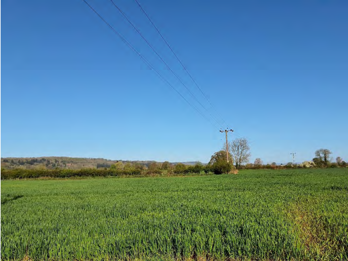
Figure 7.8: Typical view of the LCT
