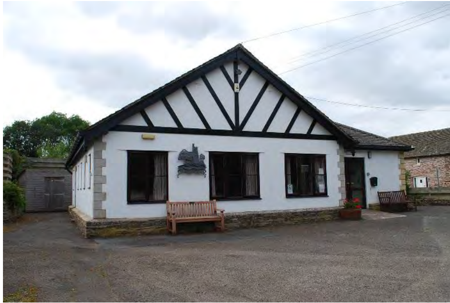
Figure 5 Staunton-on-Arrow village hall
