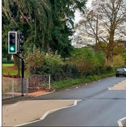
Figure 11 – Delivery of pedestrian crossing and footway at Lugwardine
