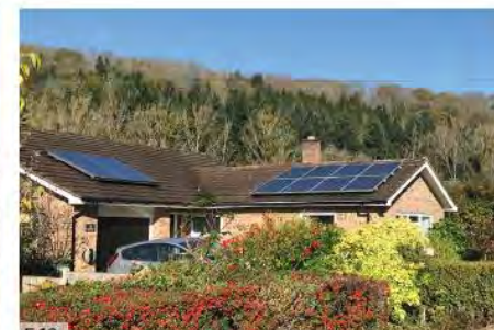
F.12 Figure 12: Bungalows within modern 1960's development Pentaloe Close.
