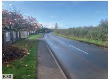
F.30 Figure 30: View south along Dormington Road.
