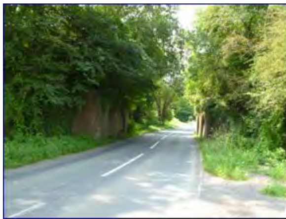
Figure 12 Former bridge over B4399
