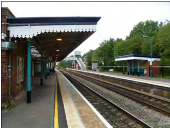
Figure 3 Leominster Station Access to Southbound Platform
