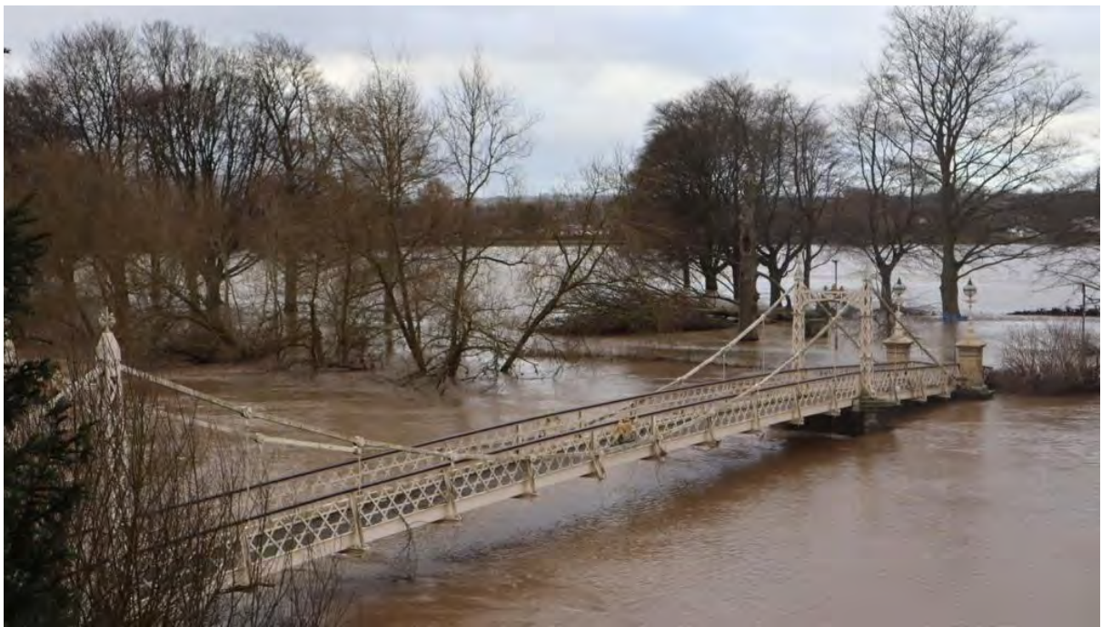
Above: Swollen River Wye at Victoria Bridge, Hereford © Herefordshire Council Front cover image: Flooding in the centre of Hereford © Herefordshire Council
