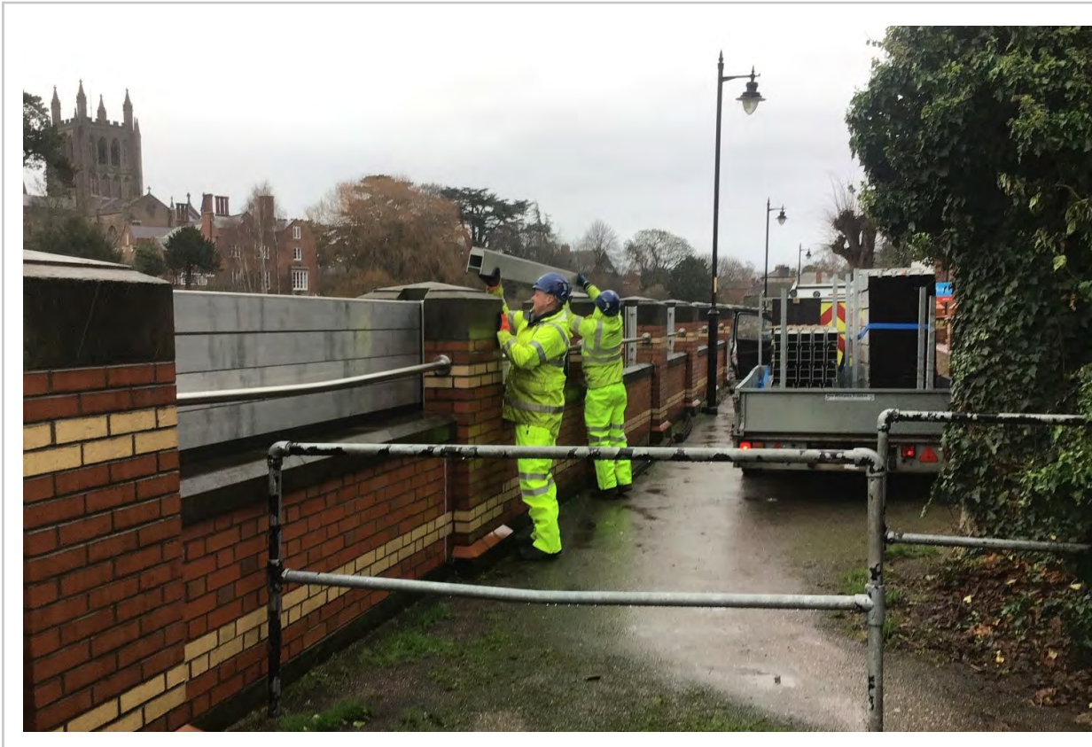
Flood defences being erected © Herefordshire Council
