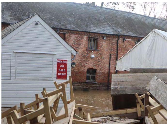
Photo: Storm damage in Herefordshire © Herefordshire Council
