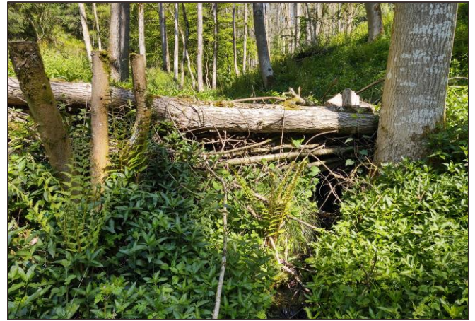
FIGURE 4 LEAKY DAM AT CROFT CASTLE, 5 MONTHS LATER
