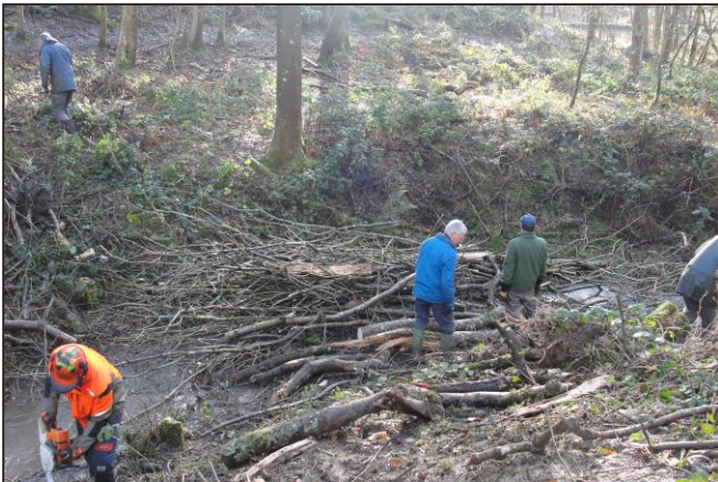
FIGURE 3 NATIONAL TRUST VOLUNTEERS AND STAFF BUILDING LEAKY DAMS IN FISHPOOL VALLEY
