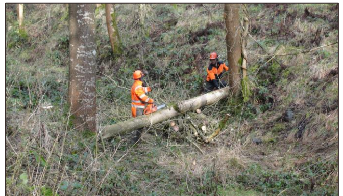
FIGURE 5 PROJECT PARTNERS USING EXISTING TREES TO WEDGE LEAKY DAM
