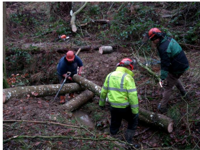
FIGURE 2 PROJECT PARTNERS WORKING TOGETHER TO BUILD LEAKY DAMS AT CROFT CASTLE
