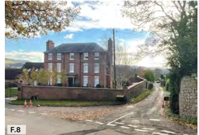
Figure 08: Grade II listed Stone House.
