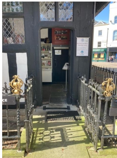
Image of step at St Peter's Street entrance
