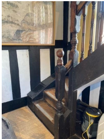
Image of the stairs as they turn
