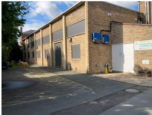
Image of disabled car parking spaces at front of building
