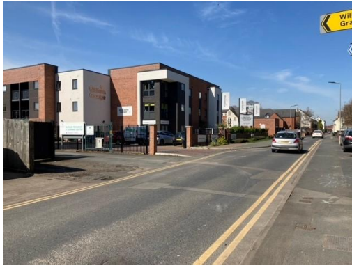
Image of entrance from Friars Street
