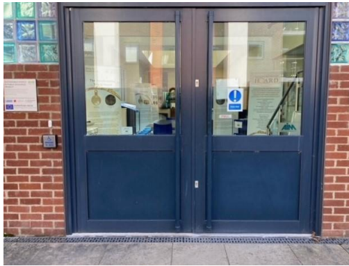
Image of entrance doorway
