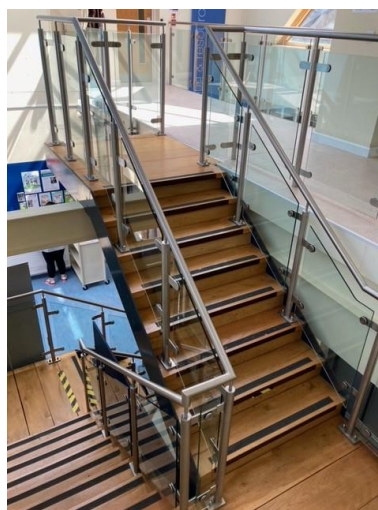
Image of the stairs at the first floor
