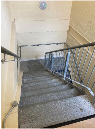
Image of the first run of stairs and the platform
