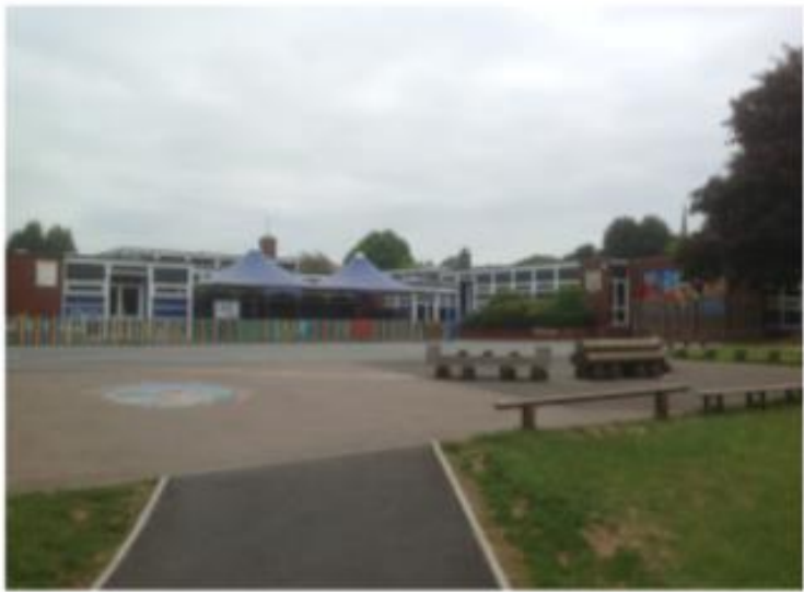
Ashfield Park Primary School
