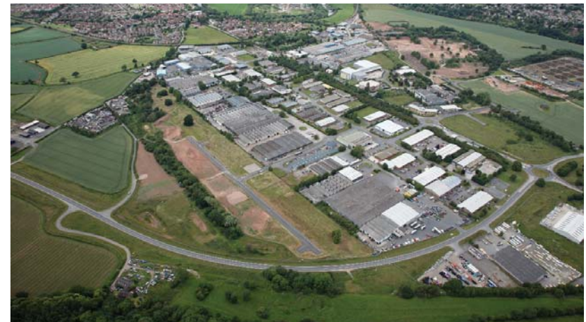
Figure 1.3 Hereford Enterprise Zone at Rotherwas, Hereford
