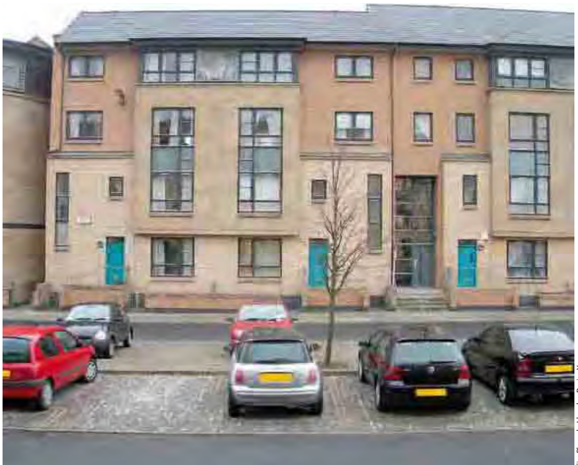
Figure 8.9 An example of on-street parking in the centre of the street that helps to separate the car from other users and provides strong surveillance of the cars.
