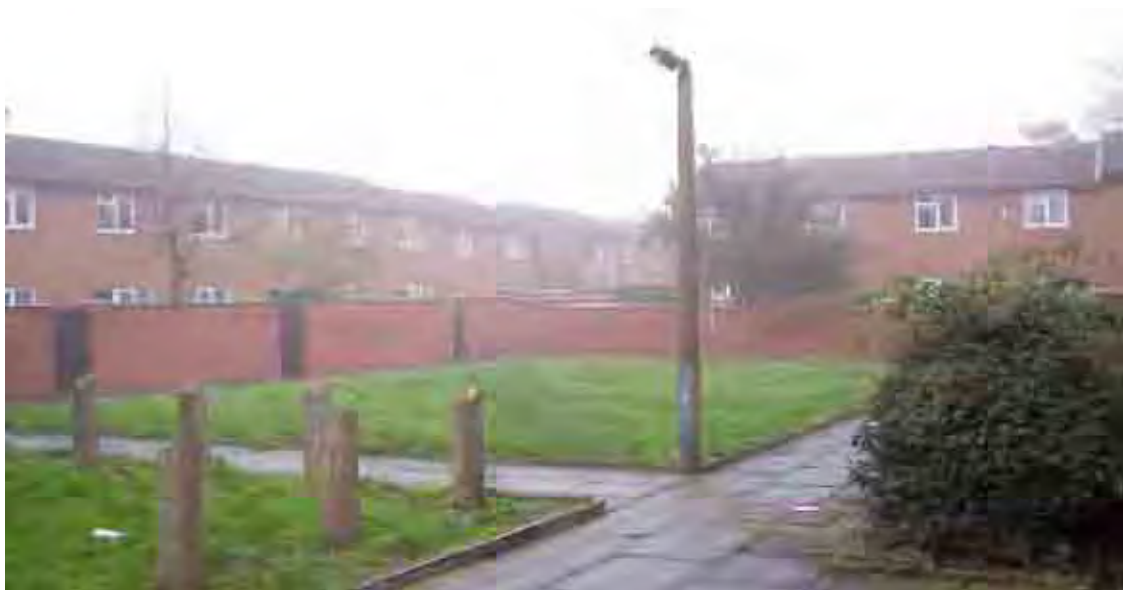
Figure 2.2 A poor-quality space with a layout where pedestrians and vehicles are segregated. It has not been a success and the area is now undergoing regeneration.
