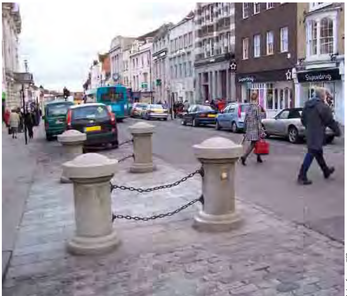
Figure 6.2 Informal crossing, Colchester – although the chains and a lack of tactile paving are hazardous to blind or partially-sighted people.
