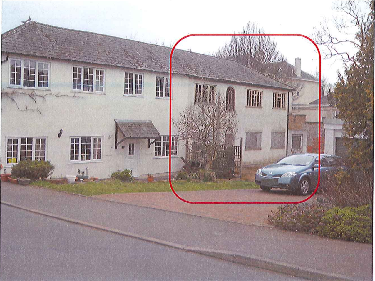
Photos of the front of property taken March 2012
