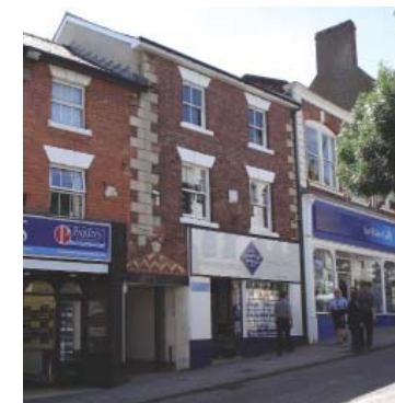
Late C20 shop front imposed on an earlier building
