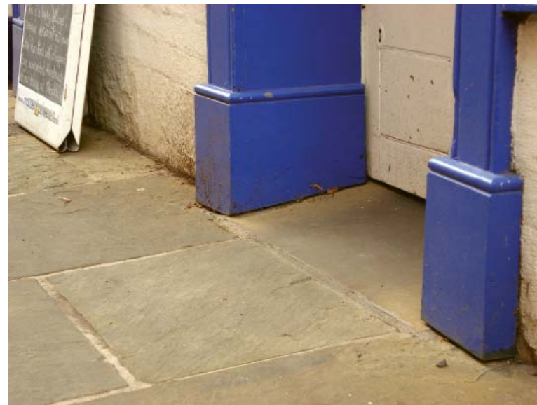
Pavement ramped slightly to ease access into the shop door
