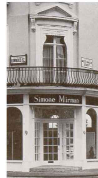
An example of a sympathetically designed C20 shop front which replaced unsuitable plate glass windows
