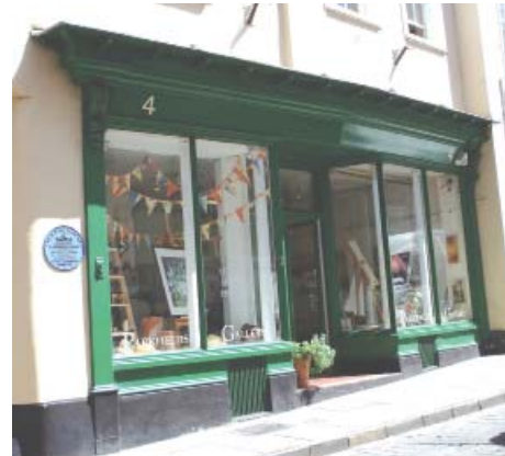
Recess doorway and deep glazing bars project light and shadow over shop front
