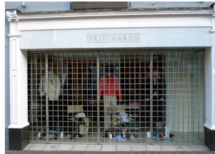
This grille is set behind pilasters and is removable
