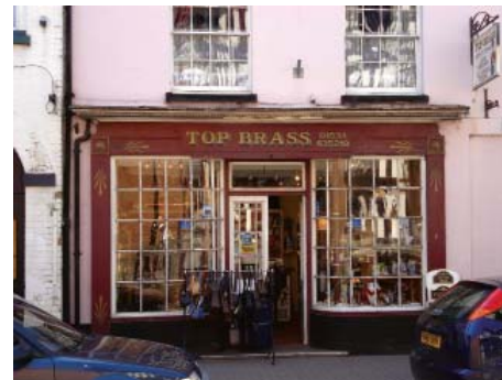
A late C18/early C19 shop front in Ledbury with deep entablature.
