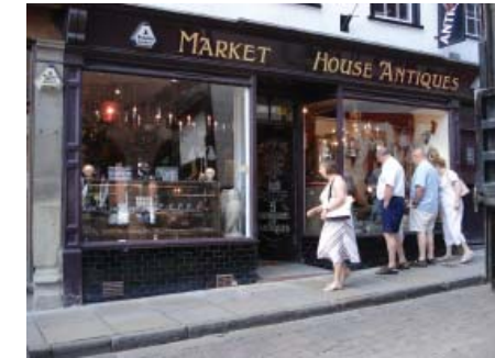
Victorian shop front in Ross with console brackets and plate glass windows
