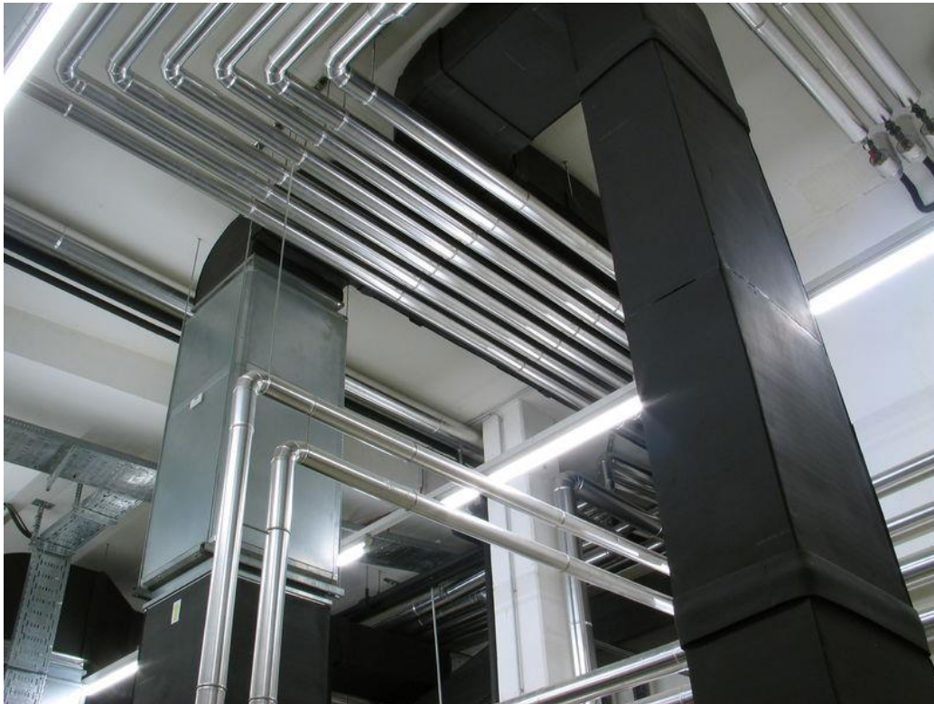
Figure 17: Example of a heat network
