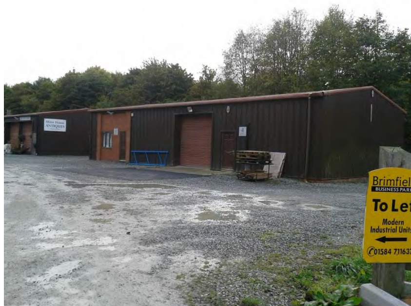
Industrial units, Brimfield
