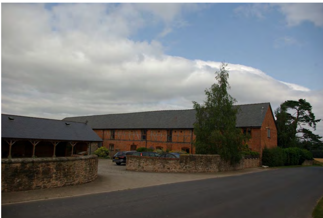
Merry Hill Farm Barn – residential barn conversion
