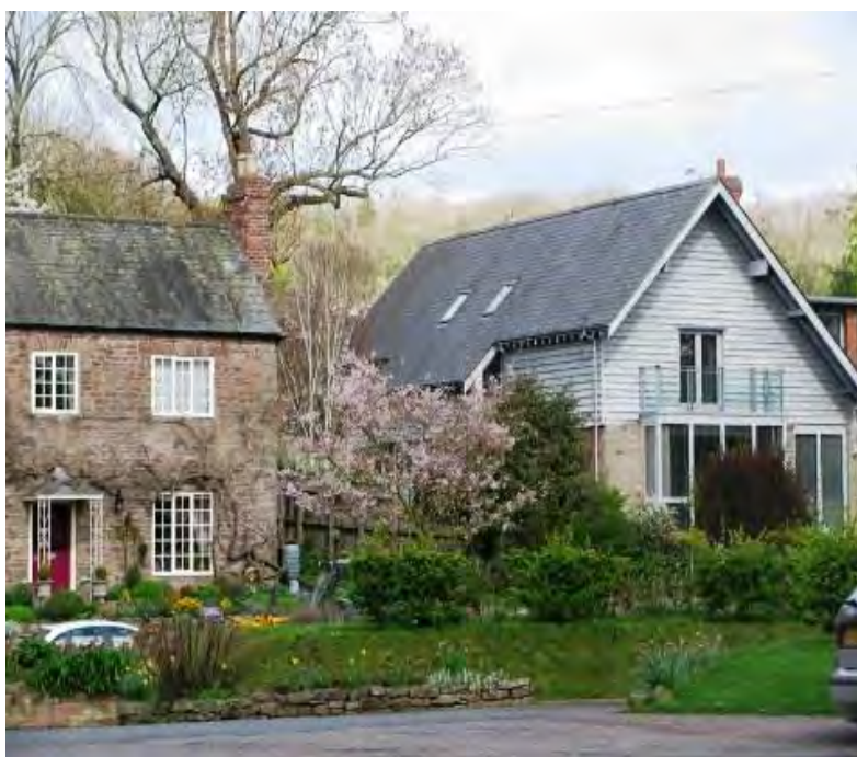
Old and New designs meet on this infill site in the Conservation area
