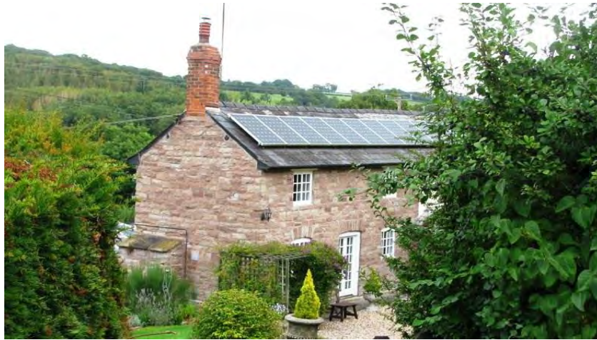
Keel House Panels on the roof
