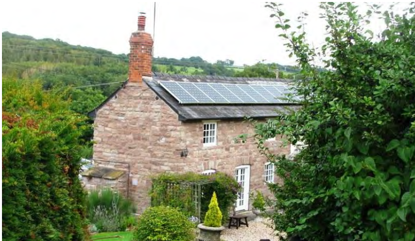
Keel House Panels on the roof
