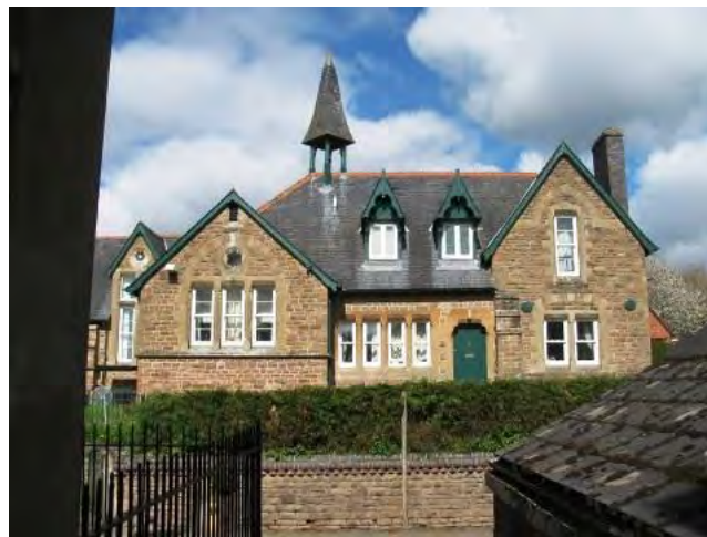
The Old School meeting housing needs
