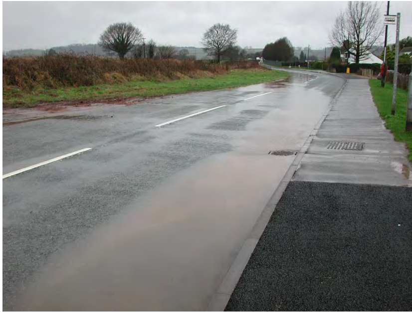
Flooding near Doctor's Surgery, B4349 Feb 2002
