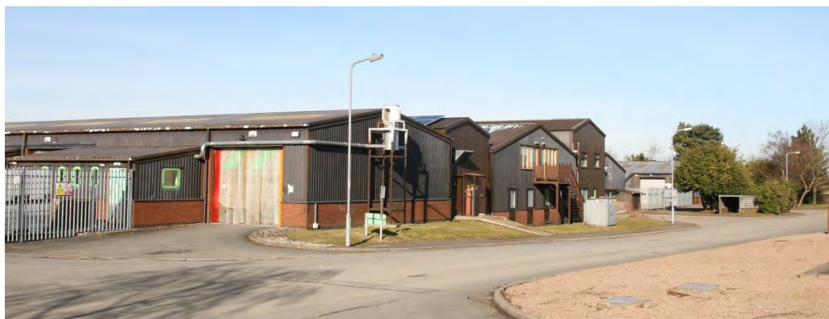
Gooses Foot Industrial Estate
