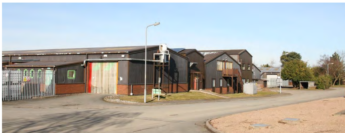
Gooses Foot Industrial Estate
