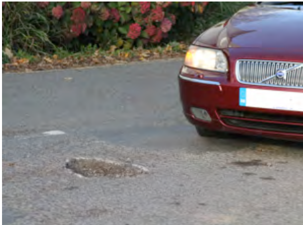
Main Access Road into the Village from the A44
